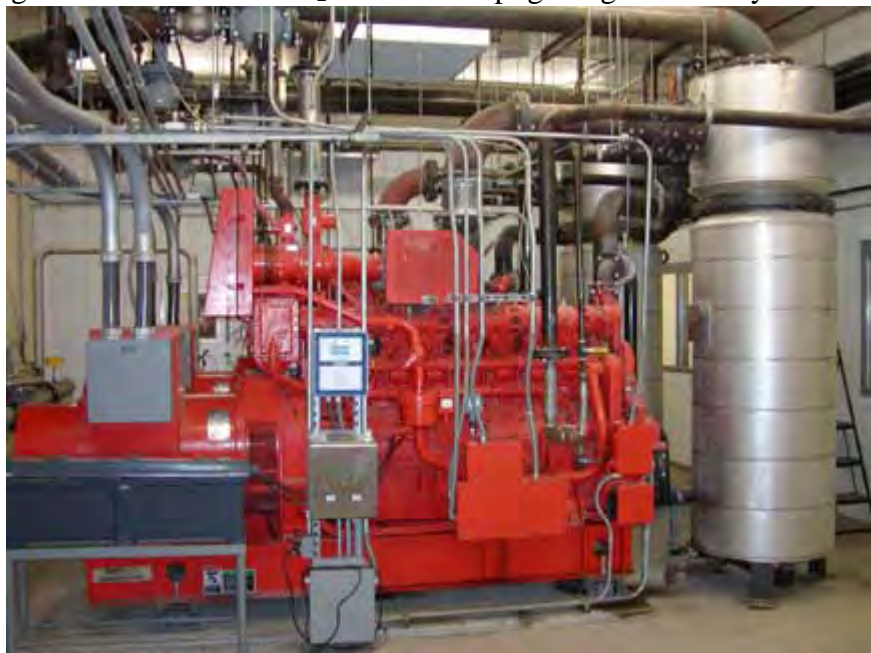
Photo: Ag Environmental Solutions, LLC
