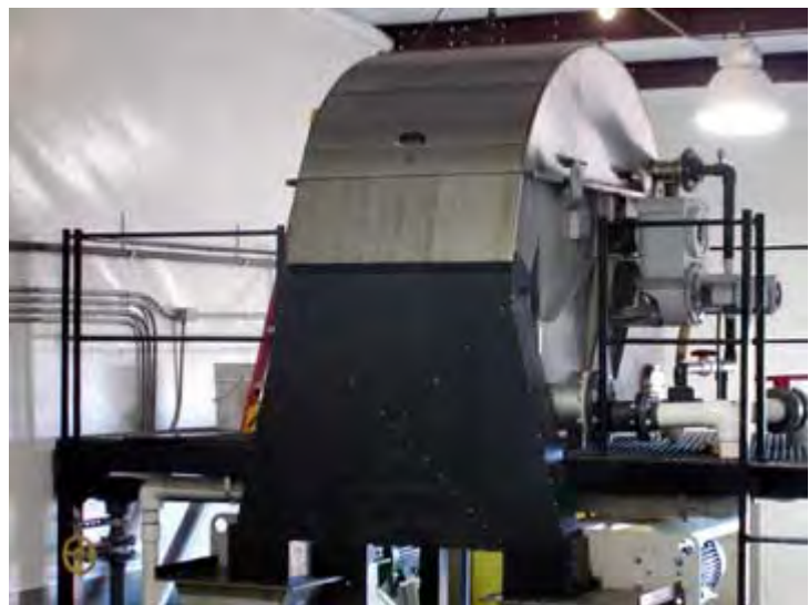
Photo: Ag Environmental Solutions, LLC
